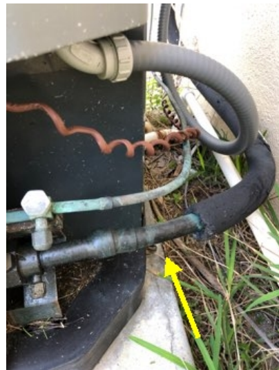
Refrigerant Line Missing Insulation
