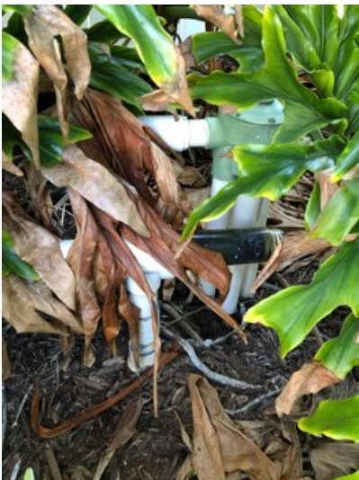
Sprinkler System Filter
