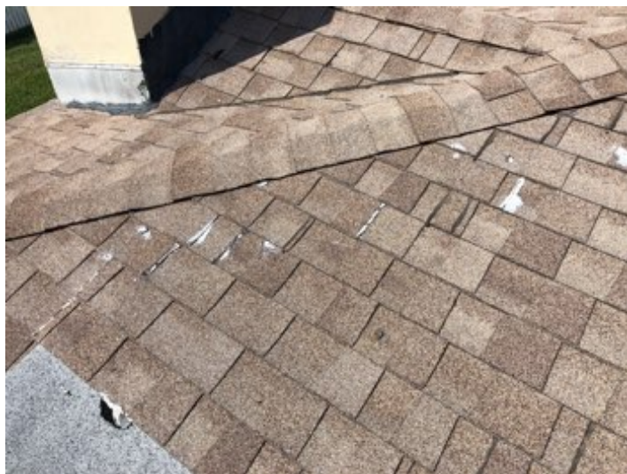
Previous Shingle Repairs w/ Caulk or Sealant
