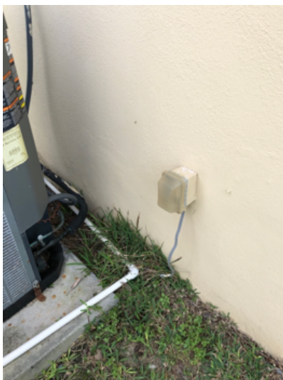
Outdoor Outlet Improperly Installed
