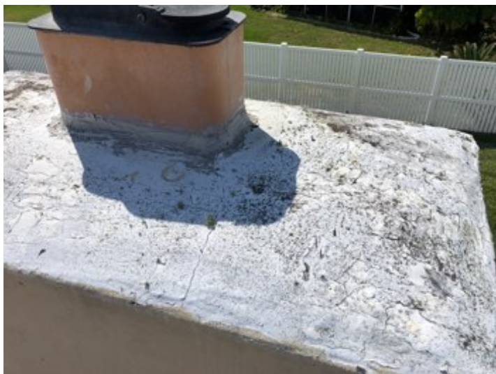
Recommend Sealing or Masonary Repair
