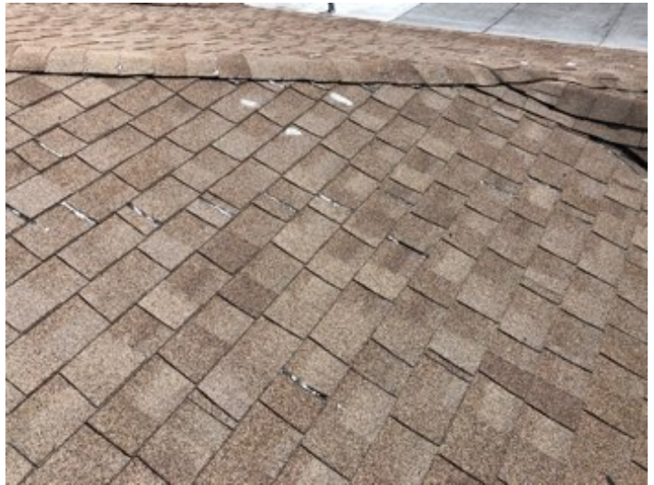
Caulking or Silicon from Previous Repair
