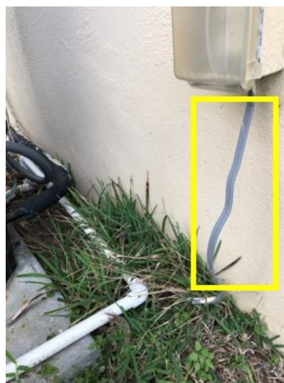
Wire Should Be in Pipe
