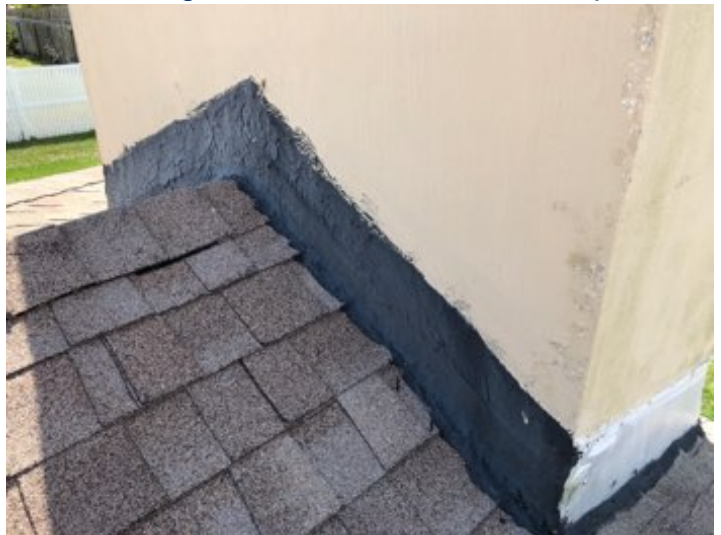
Heavy Tar Where Flashing Should Be
